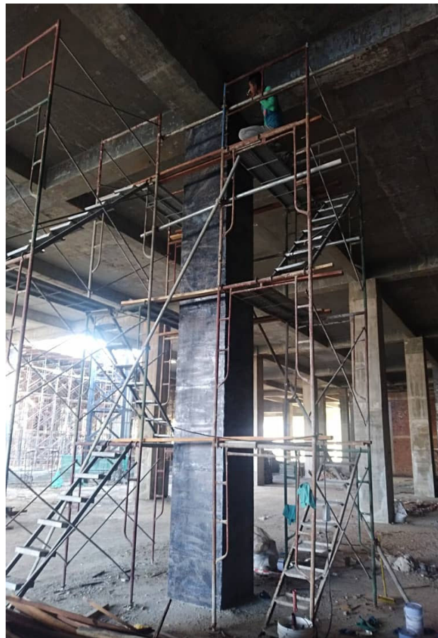
Build Wrap Pro 300 apply on Column
