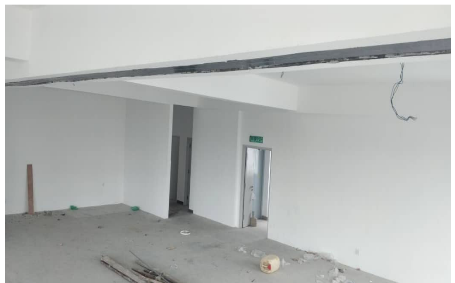
“Build Strip STD 1030” Installed at Reinforced Beam [2 nos Strip]
