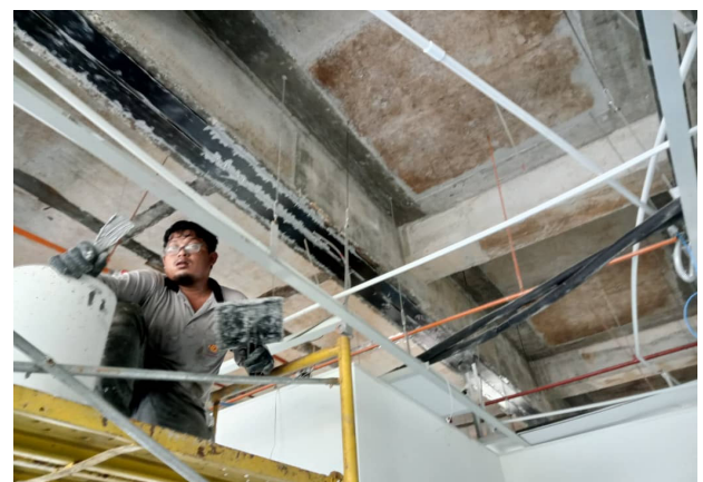
Build Strip Pro 1030 [2 nos Strip at Beam]
