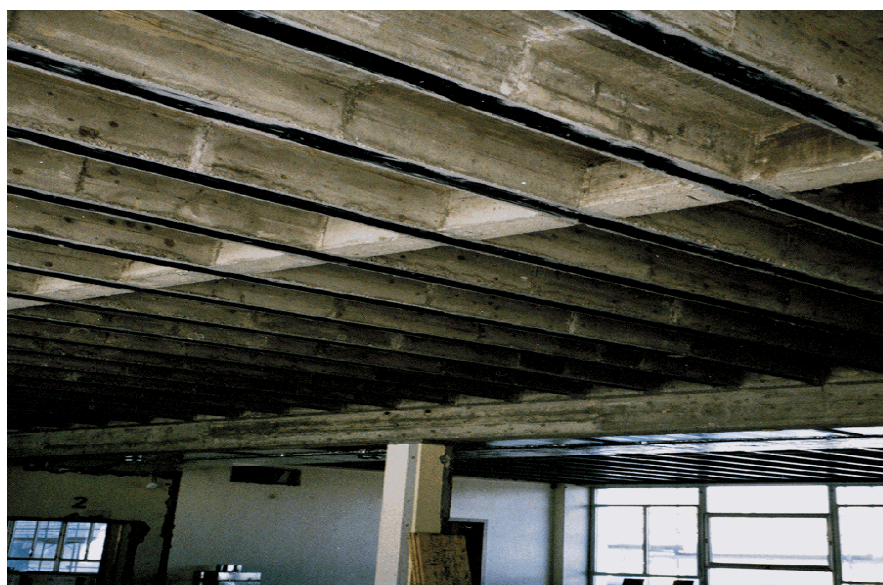
“Build Strip HS” Installed at Reinforced Beam
