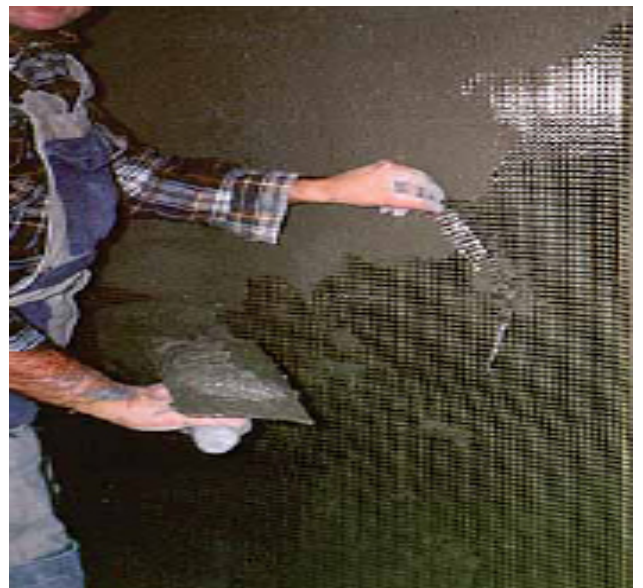
Install on Build Mesh CF 30010 on Wall
