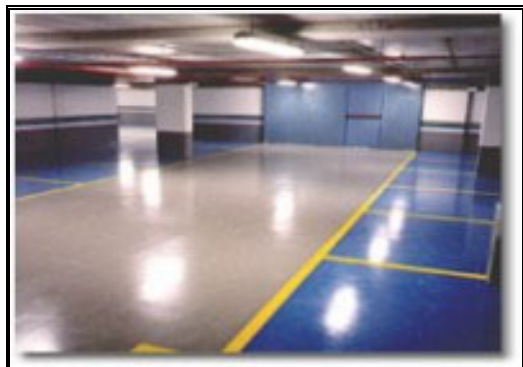
Pharmaceutical Processing Floor
