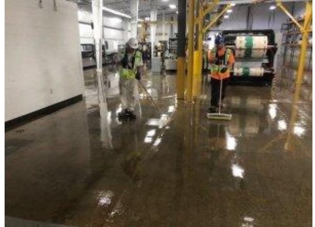
Lamco Coat 6290C Apply on Industrial Flooring
