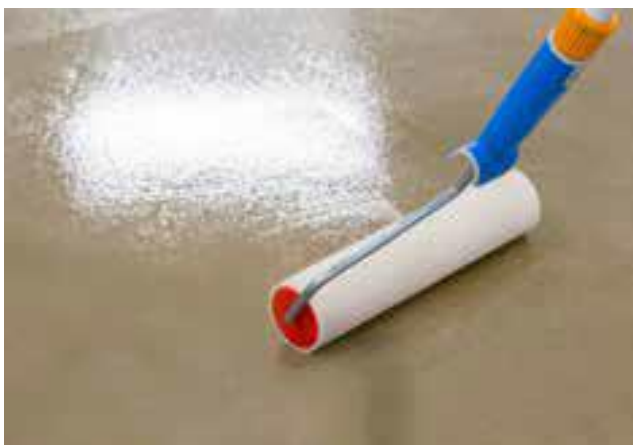
Lamco Coat 6290C Apply by Roller
