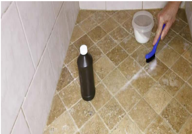
Washing the existing floor tiles joint
