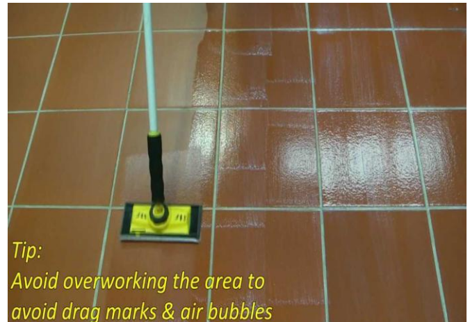
Apply Lamco Coat 6290C on floor joint
