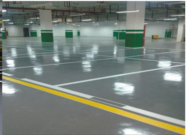
Lamco Coat 6290C Apply on Car Park Floor Primer Coat with Color, Body Coat with Color & Top/Finish Clear Coat [Matt & Glossy]
