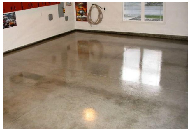
Apply Lamco Coat 6290C on Floor
