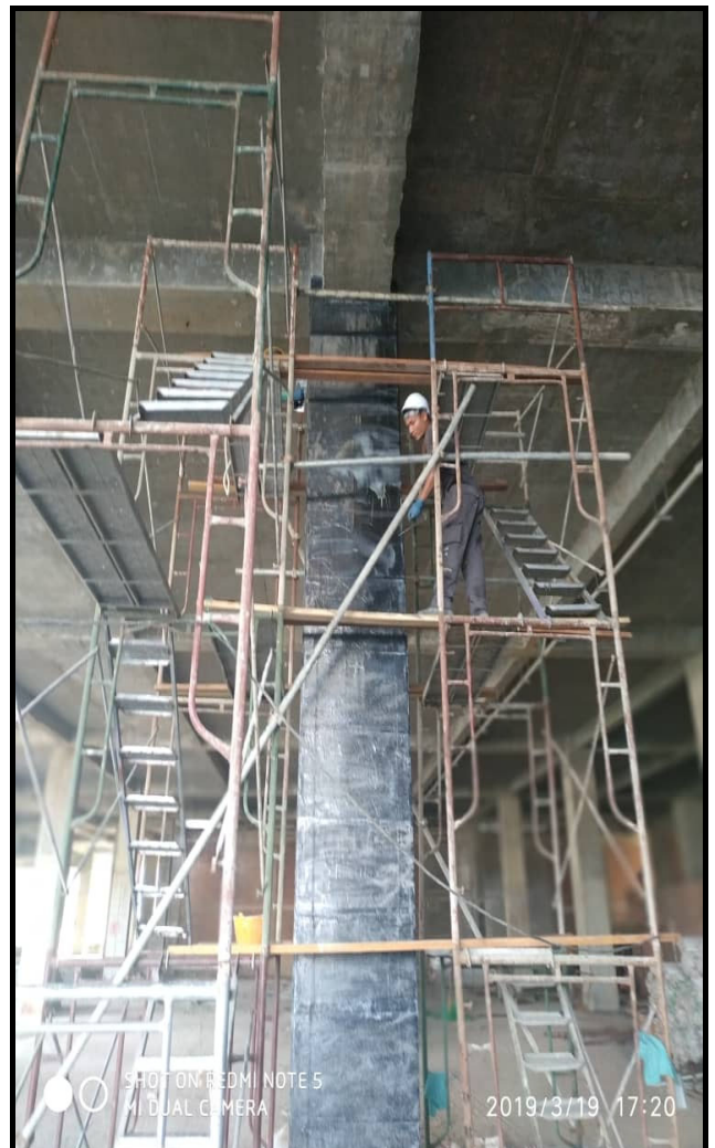
Build Wrap HS 300 apply on Column
