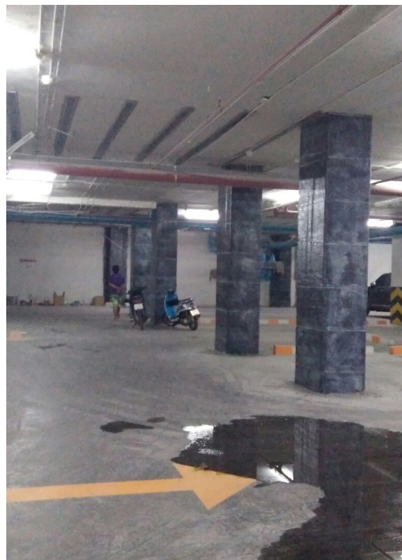
Build Wrap HS 300, apply on Column
