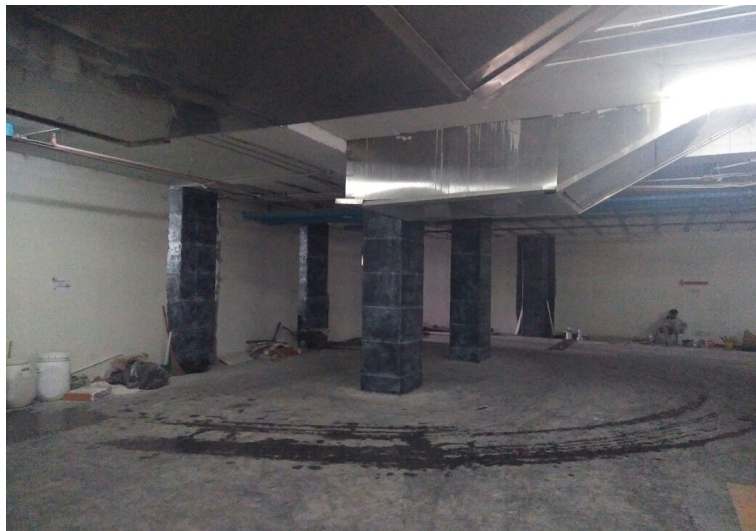
Build Wrap HS 300, apply on Column
