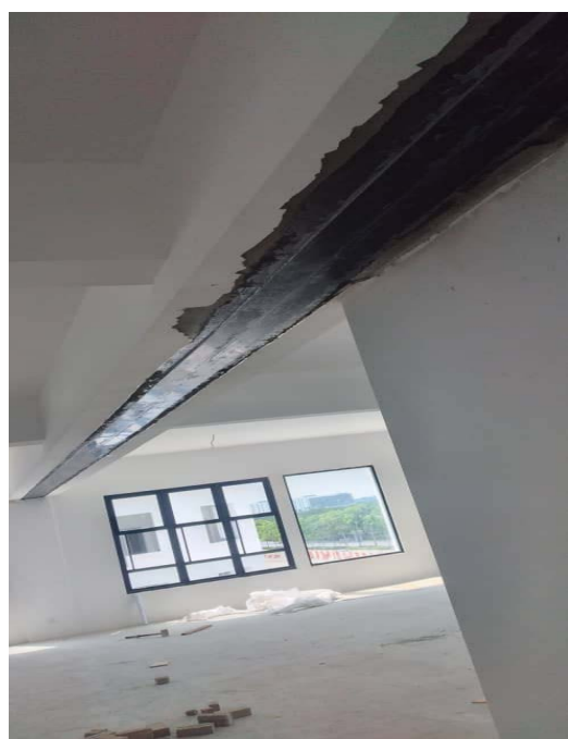
“Build Strip STD 1030” Installed at Reinforced Beam [2 nos Strip]
