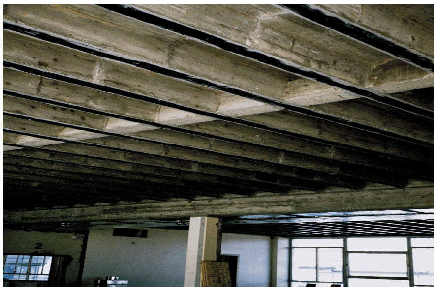
“Build Strip HS” Installed at Reinforced Beam
