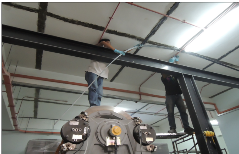
Build Strip HM 1014, apply on Slab
