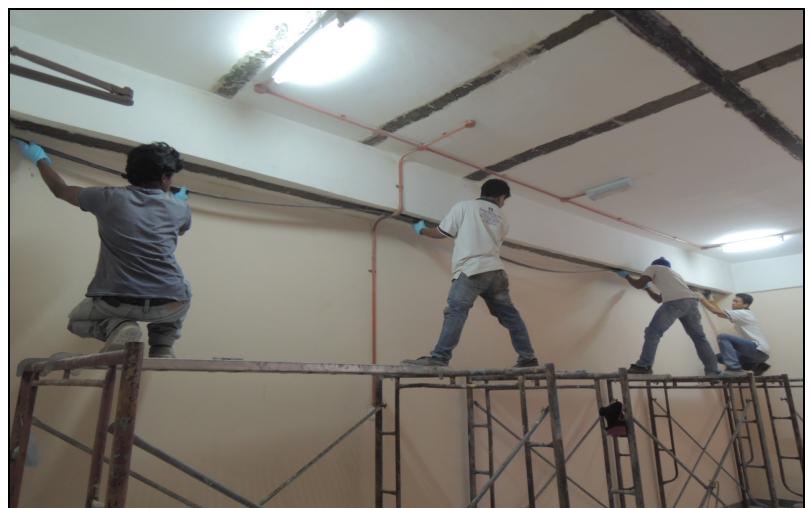
Build Strip HM 1014, apply on Beam
