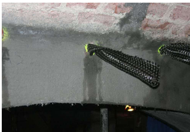
Install of Build Mesh CF on Void Holes
