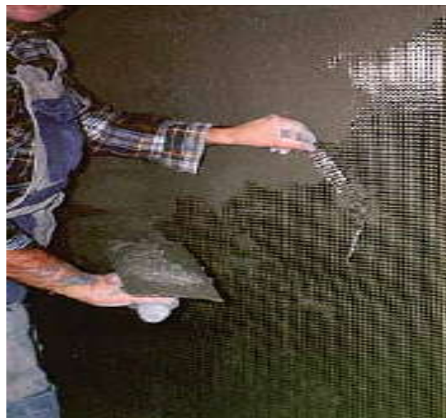
Install on Build Mesh CF 30020 on Wall
