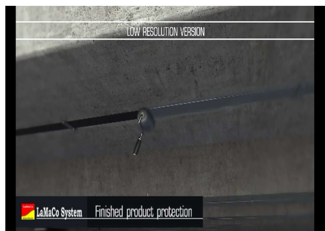
18] Fireproofing Protection on Build Strip PB
