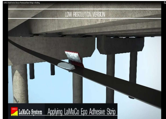
14] Laying the LaMaCo-Epo Adhesive Strip
