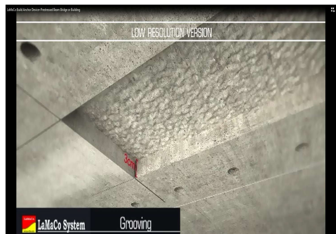
4] Hack Out or Grooving, Depth Set 30mm
