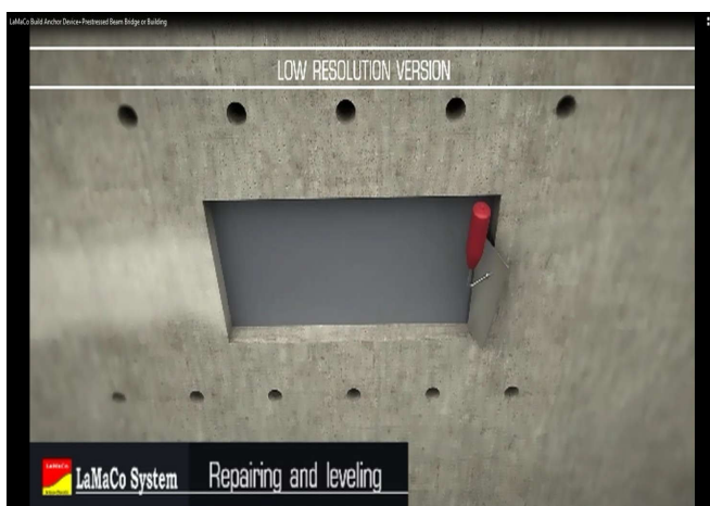
5] Patching to Leveling
