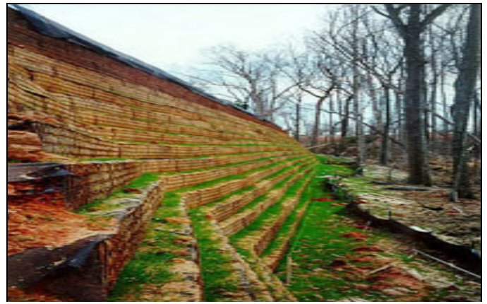
“LaMaCo Progrid BXPET” install on Slope Step
