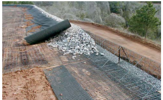
“LaMaCo Progrid UXPP” install on Side Retaining Wall & Main Street Way
