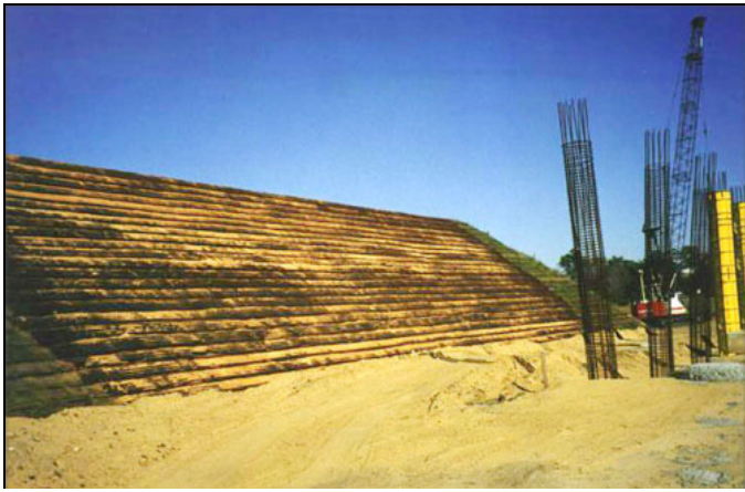
“LaMaCo Progrid BXGF” install on Slope Step
