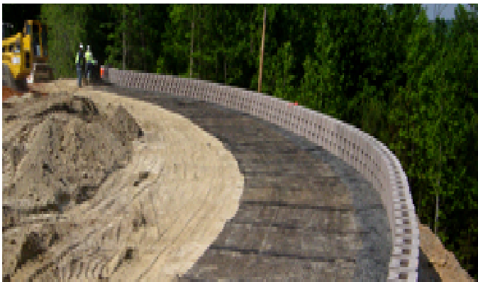
“LaMaCo Progrid UXPP” install on Side Retaining Wall
