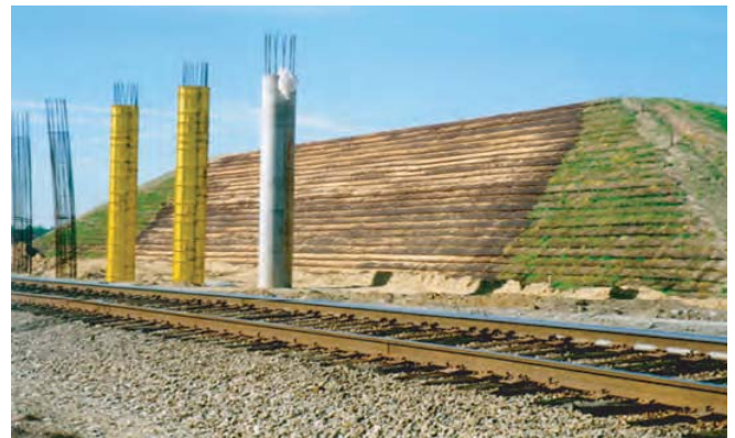
“LaMaCo Progrid UXPP” install on Railway Side Retaining Wall
