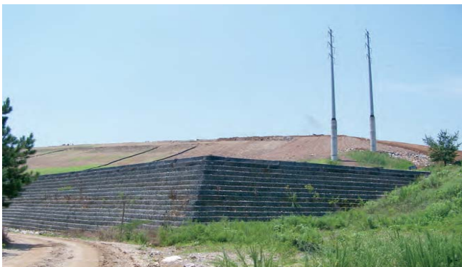
“LaMaCo Progrid BXPET” install on Side Retaining Wall
