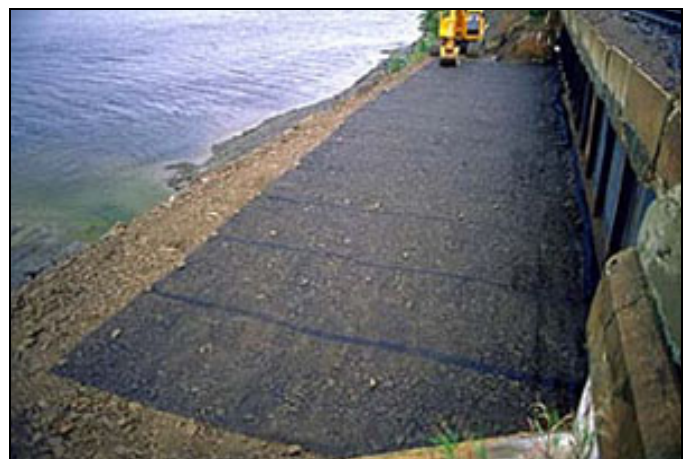
"LaMaCo Progrid BXPP" install on Sea Landfill
