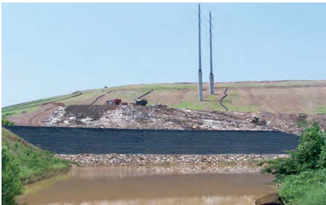
“LaMaCo Progrid BXPET” install on Side Retaining Wall & Main Street Way
